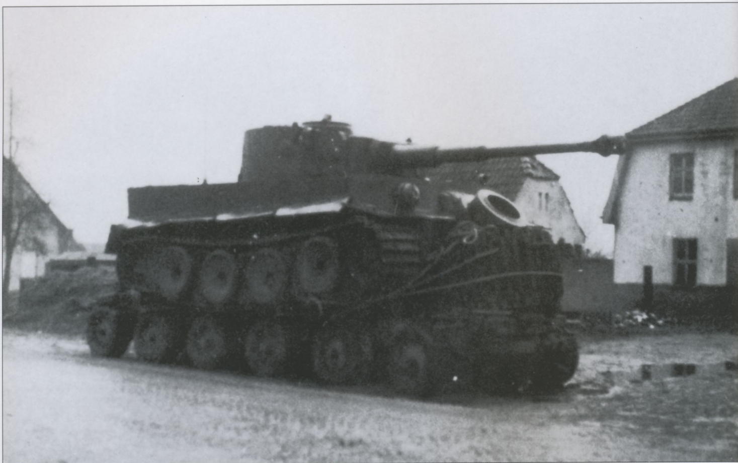
This early Tiger I was captured in Germany by the British Army and shipped to England for evaluation after the war. It has been fitted with the narrow transport tracks and is seen loaded on a Gotha 80 ton transporter with the wide battle tracks coiled up on the front of the trailer.
