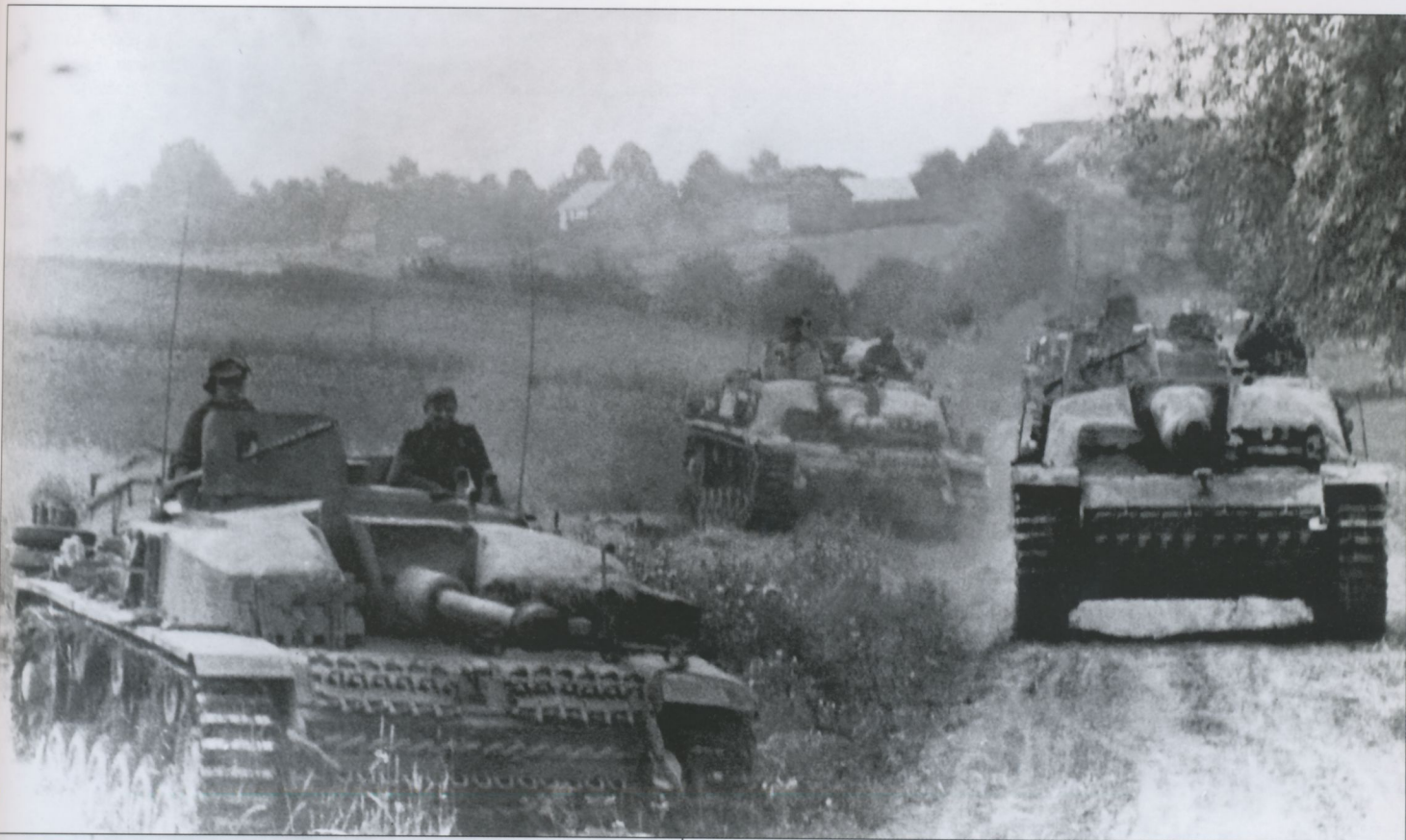
Three photos of a column of StuG.III Ausf.G somewhere on the Eastern Front in the late summer of 1944. The concrete reinforcement has been applied with an artistic flair and projects out around the driver's visor. Salvaged T-34 tracks have been hung on the spare track bracket on the front of one of the vehicles, probably because the wider track provides better protection. Usually, the Schürzen plates lapped front over back to prevent them from being snagged driving through dense brush but here they have been installed backwards.
