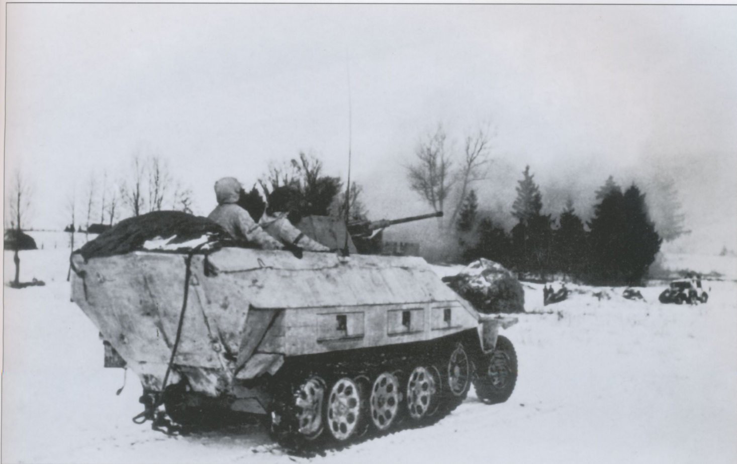
The Sd.Kfz.251/17 Ausf.D armed with a 2cm KwK38 autocannon, is rarely seen in photographs. The gun was mounted on a pedestal and a small armored, open top turret that protected the operator surrounded the upper part.
