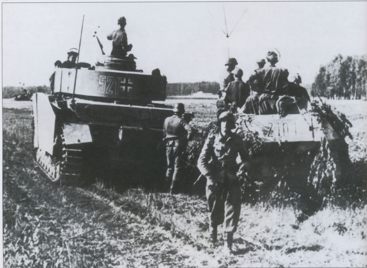
A Pz.Kpfw.IV Ausf.J with an Sd.Kfz.251/3 Ausf.C on the Eastern Front during the summer of 1944. The tactical numbers on the turret Schürzen are probably red with a white outline compared to the black center of the national cross. The Sd.Kfz.251/3 mittlere Funkpanzerwagen has a 2m Sternantenne attached to a mount on the rear plate and was used for the FuG8 radio set.
