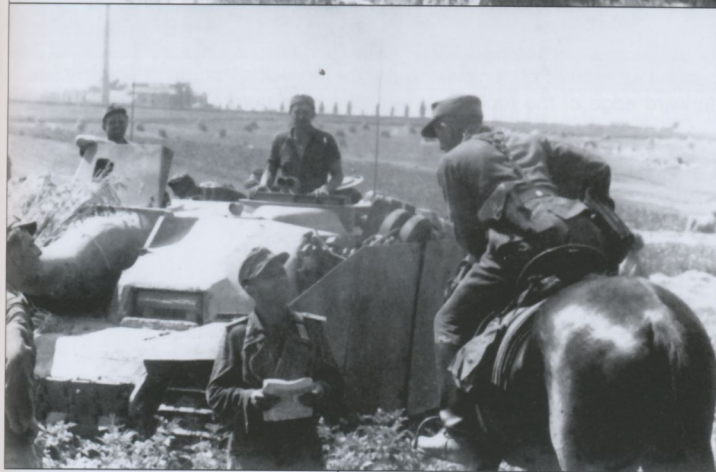
Three photos of a column of StuG.III Ausf.G somewhere on the Eastern Front in the late summer of 1944. The concrete reinforcement has been applied with an artistic flair and projects out around the driver's visor. Salvaged T-34 tracks have been hung on the spare track bracket on the front of one of the vehicles, probably because the wider track provides better protection. Usually, the Schürzen plates lapped front over back to prevent them from being snagged driving through dense brush but here they have been installed backwards.
