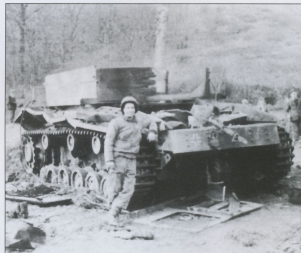
A U.S. soldier poses for a picture with a Bergepanzer III knocked out in Belgium in the fall of 1944. In January 1944, all Panzer III returned for overhaul, were ordered converted to Bergepanzer and a total of 150 were completed from March to December 1944. Although this one has been converted from an Panzer III Ausf.J, it is fitted with the early style eight-hole drive sprocket with the spacer ring to accommodate the 40cm tracks.
