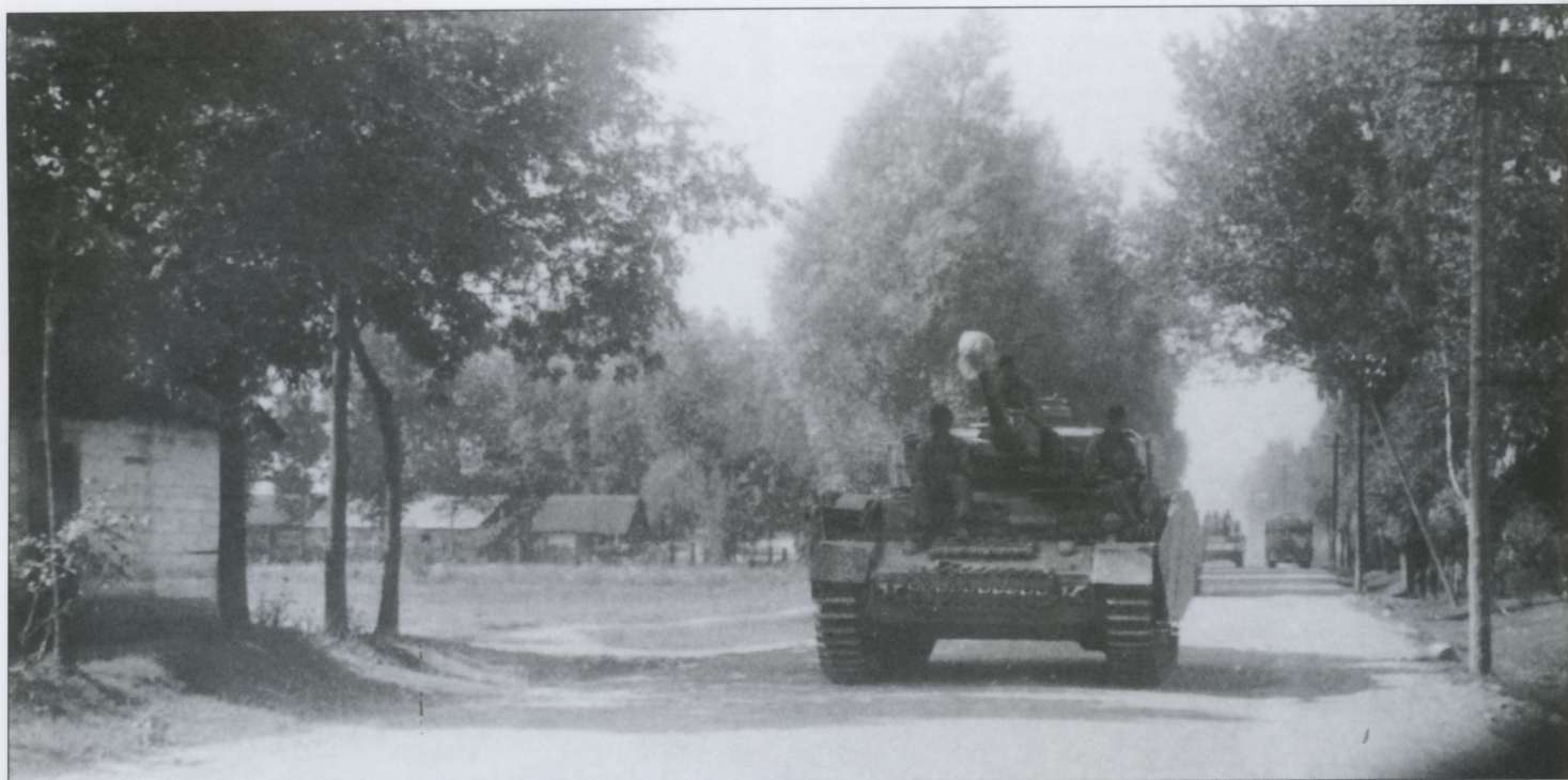
A column of Pz.Kpfw.IV Ausf.H or Ausf.J on the outskirts of an East Prussian town in the summer of 1944. They are probably new issue as there does not appear to be any battle damage and they carry a full set of Schürzen. The single Bosch headlight on the left fender is an identifying feature of the Panzer IV Ausf.H or J, as there were two headlights on the Panzer IV Ausf.G.
