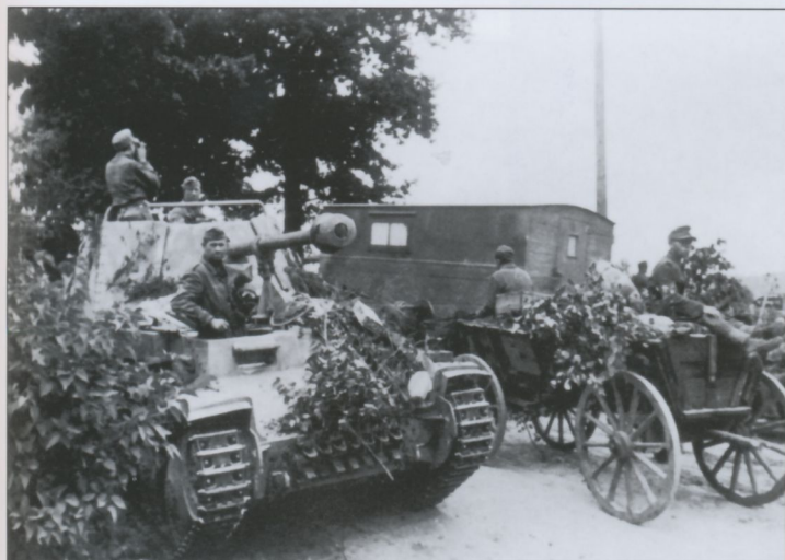
The Sd.Kfz.251/17 Ausf.D armed with a 2cm KwK38 autocannon, is rarely seen in photographs. The gun was mounted on a pedestal and a small armored, open top turret that protected the operator surrounded the upper part.
