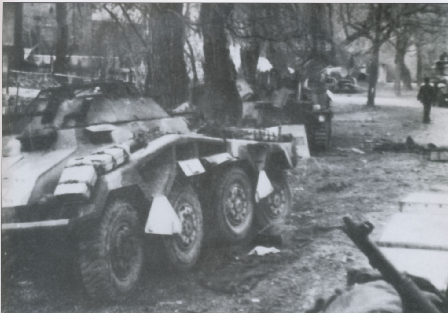
This schwere Panzerpähwagen (2cm) Sd.Kfz.234/1 sits abandoned in a German town in 1945. These heavy armored cars were issued to the Panzer-Aufklärungs-Abteilung of the Panzer and Panzer-Grenadier divisions starting in July 1944. A total of 200 were produced from June 1944 to January 1945.
