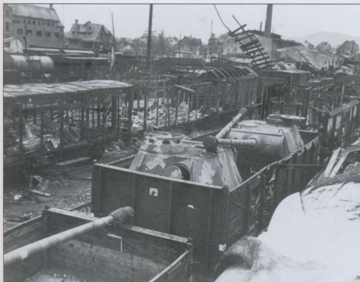
These Panther turrets were photographed in the bombed out railway station in Aschaffenburg in 1945. The turret with the colorful camouflage paint scheme is probably an Ausf.A production as it has the Nahverteidigungswaffe on the right rear of the turret roof but is lacking the Pilze socket. The other turret is obviously from an Ausf.D.
